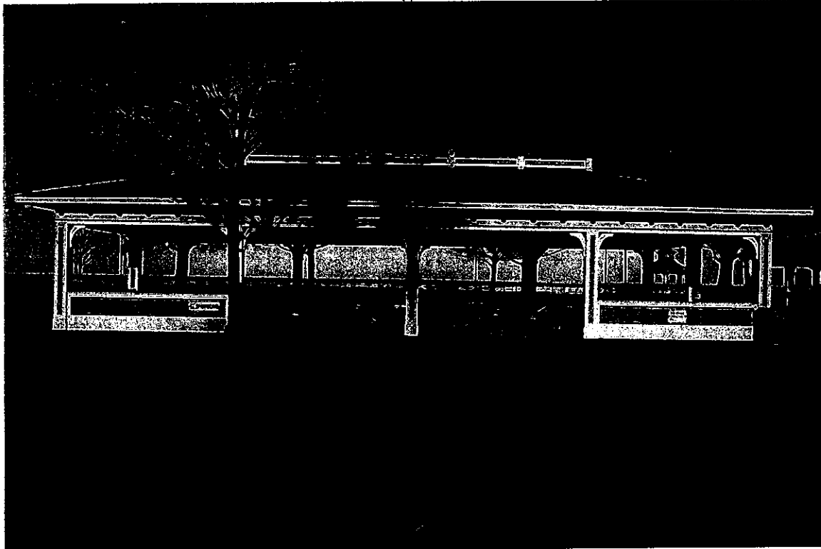
Photograph 28. Picnic Pavilion (Structure 60) in Ontario Beach Park, looking north.
