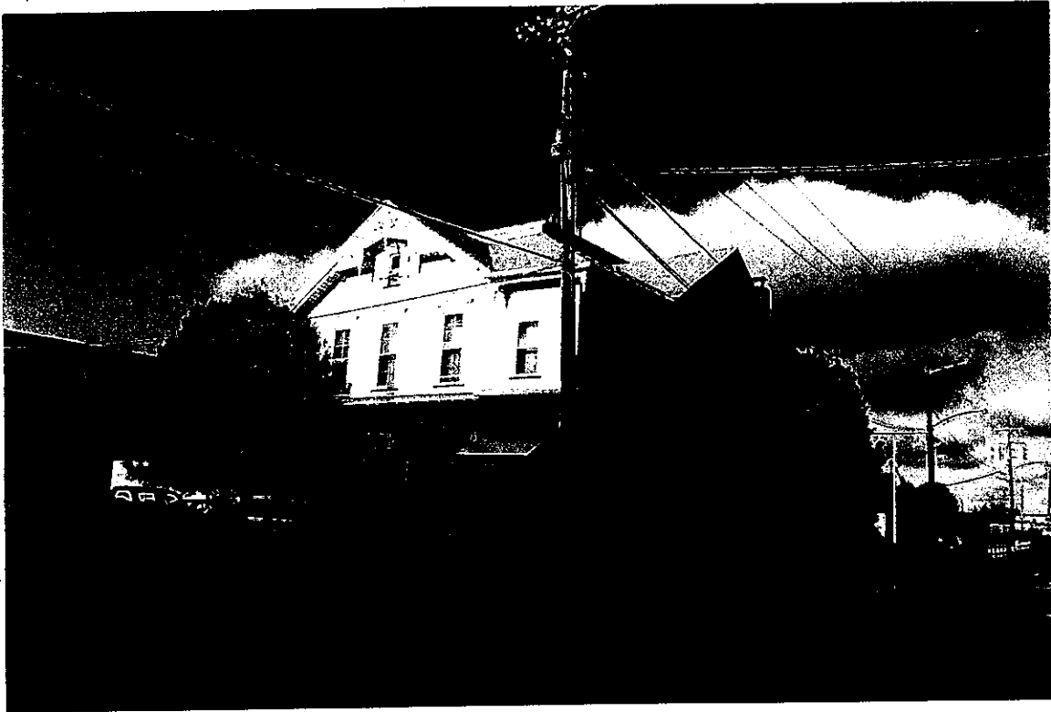
Photograph 33. Tapecon Office/1902 U.S. Customs House (Structure 23), 10 Latta Road, Potentially NR-Eligible, looking northwest
