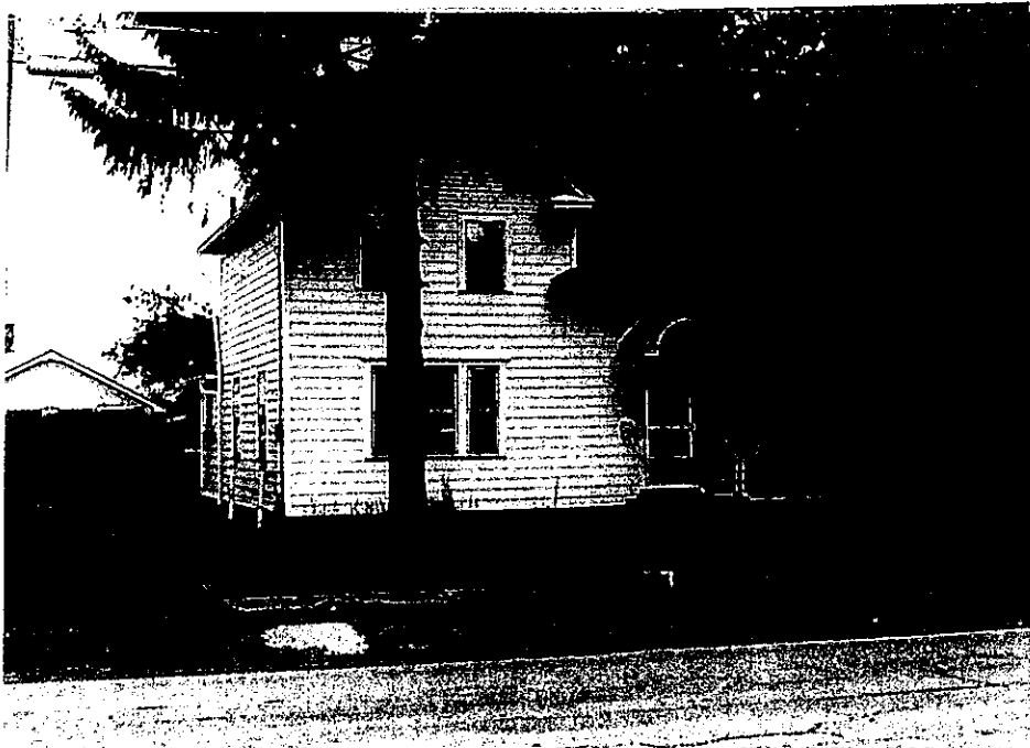
Photo 134 Structure 108, Facing southeast
