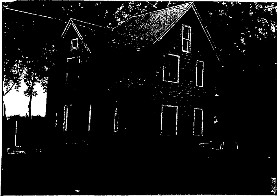
Photo 60 Structure 24 302 River Street Facing Southeast
