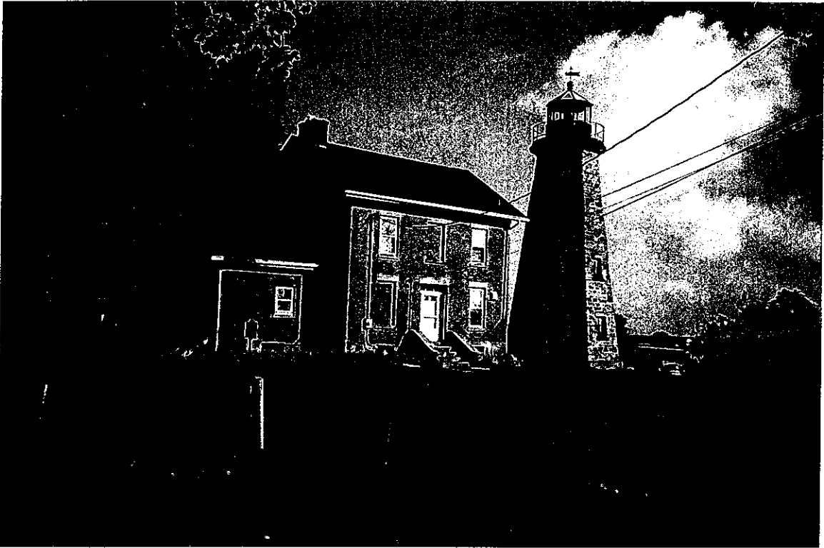
Photograph 19. The Genesee (Charlotte) Lighthouse constructed in 1822 and the Second Keeper's House constructed in 1863, from the north end of Lighthouse Street, looking north.
