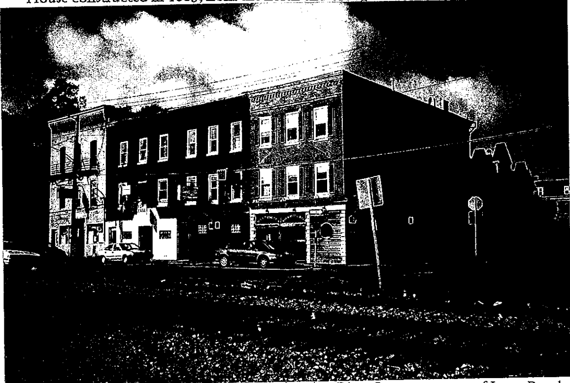
Photograph 20. Commercial Buildings at 419-431 River Street at corner of Latta Road, constructed between 1870-1900, looking southwest.
