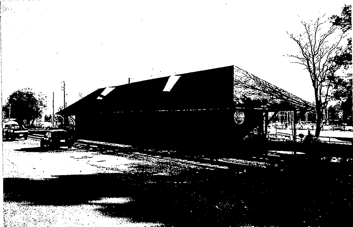
Photograph 22. The New York Central River Street (Charlotte) Station built in 1902, from River Street, looking northeast.
