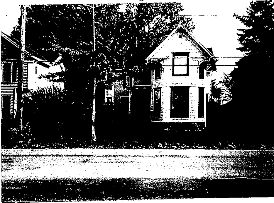
Photo 136 Structure 110, Facing east
