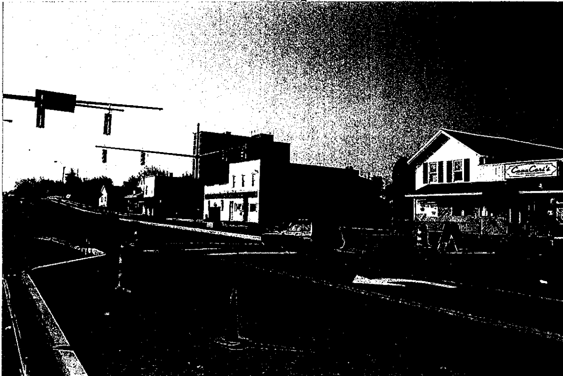
Photograph 12. General Project Area - Lake Avenue from 4653 Lake Avenue, looking south.
